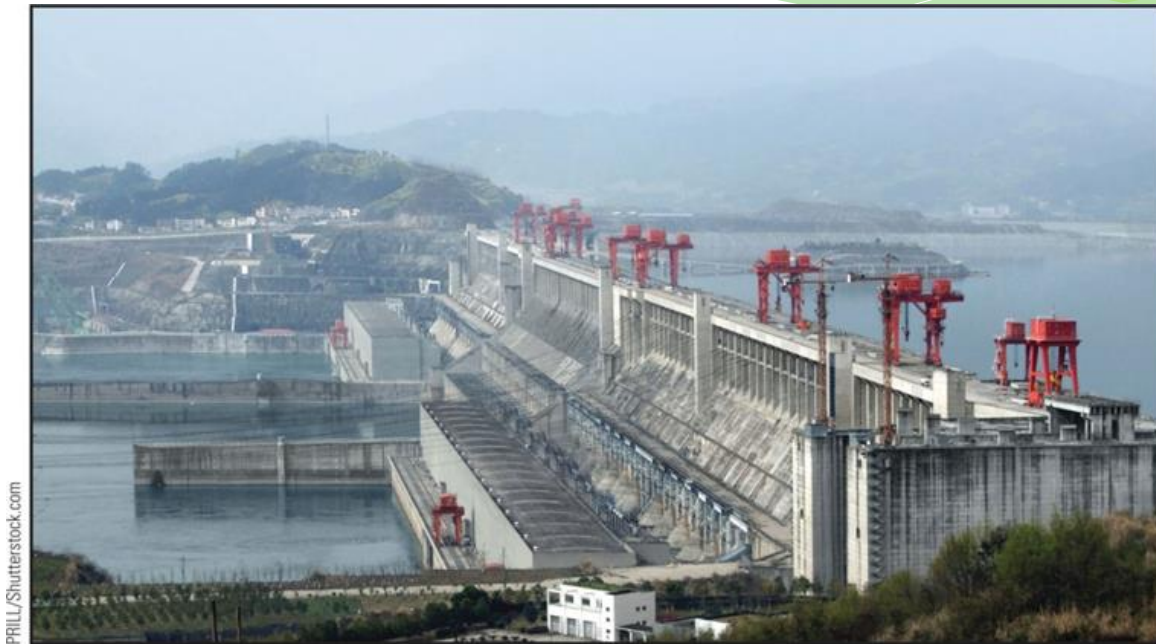
Figure 11.2: Three Gorges hydroelectric facility in China. This is the world's largest hydroelectric facility, currently rated at 22,500 MW e . The environmental consequences of the Three Gorges Dam are discussed in Energy Extra 11.2.
