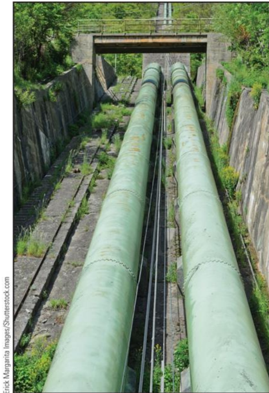
Figure 11.15: Penstocks used to divert part of a river's flow through a generating station.
