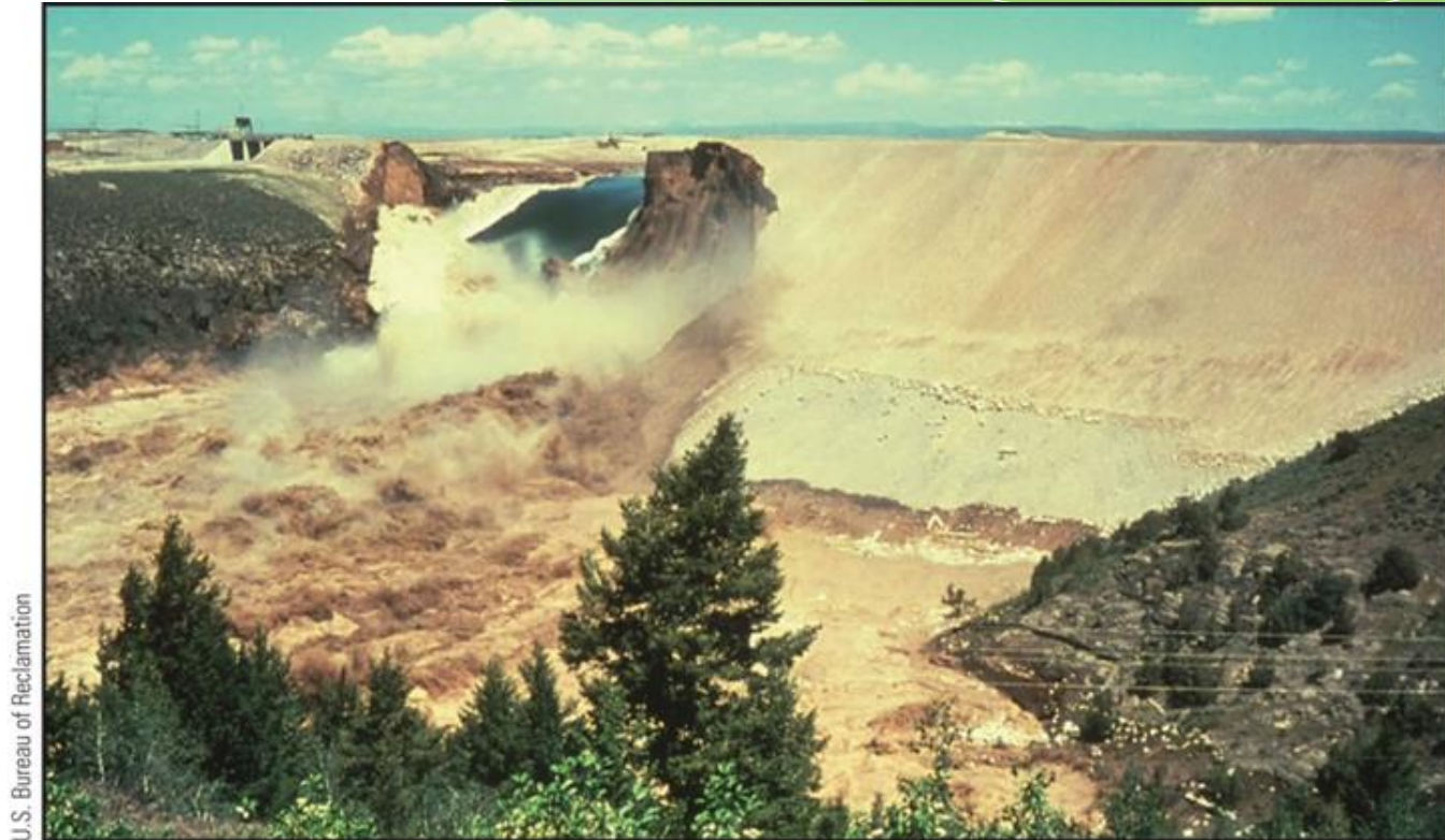
Figure 11.25: Failure of the Teton Dam in Idaho in 1976.
