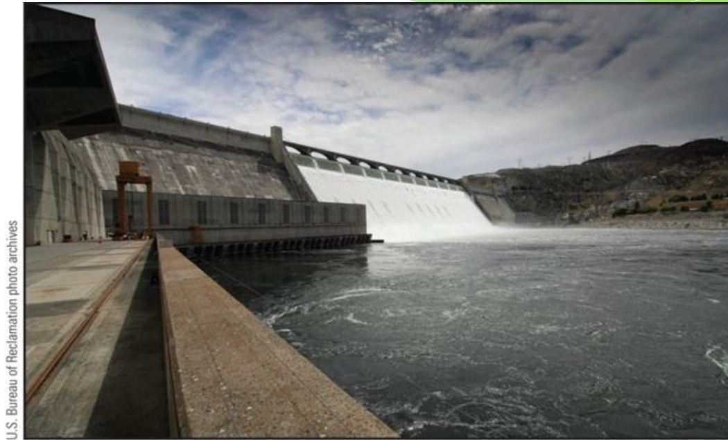
Figure 11.11: Grand Coulee Dam in Washington State, United States.
